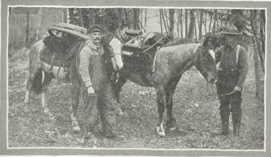
Two pumping outfits carried on two pack horses
