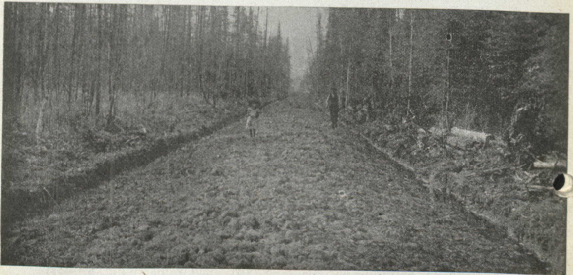
A Government Roadway in Northern Ontario in Process of Construction.
