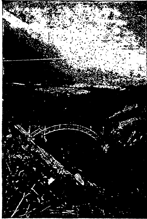
STONY CREEK BRIDGE.
