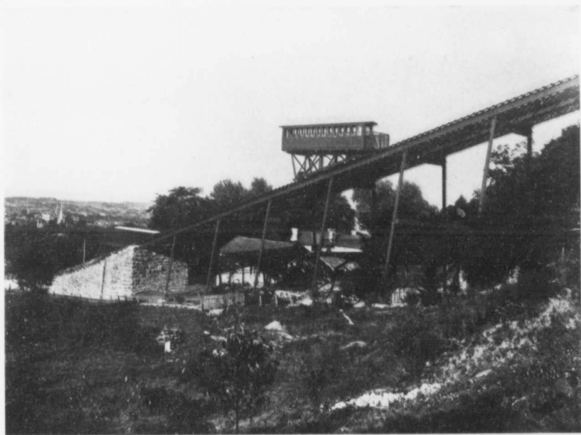
JAMES STREET INCLINE
