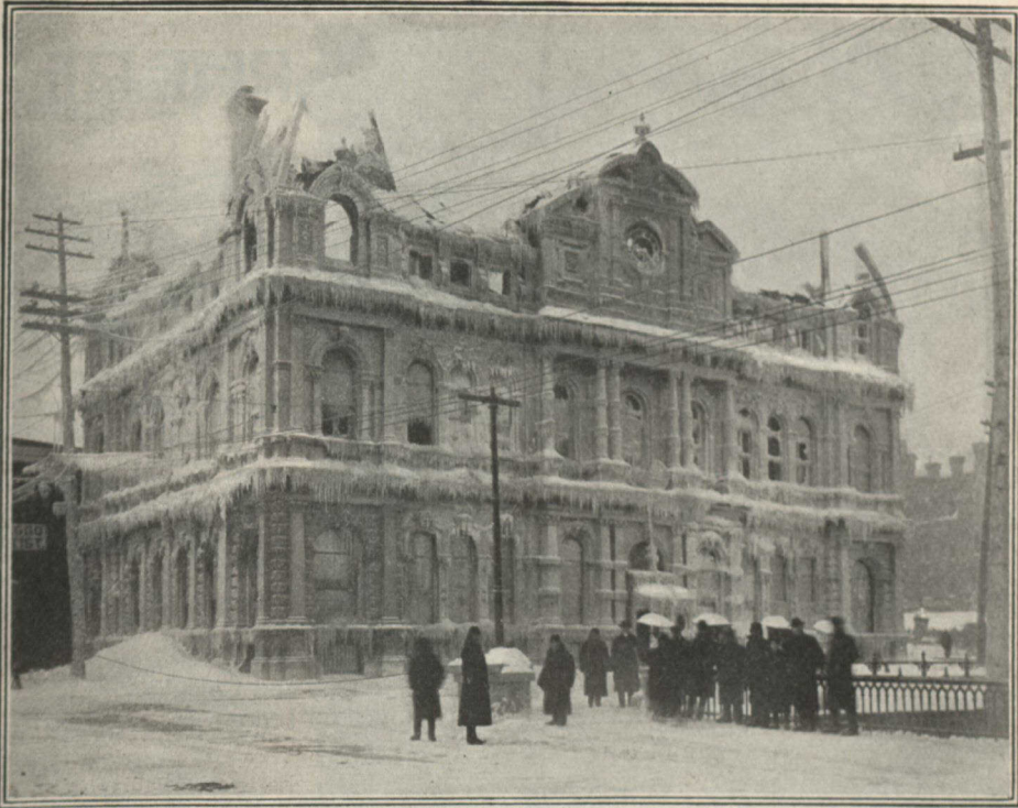
THE OTTAWA GENERAL POST-OFFICE—DAMAGED BY FIRE LAST MONTH PHOTOGRAPH BY A. J. PITTAWAY
