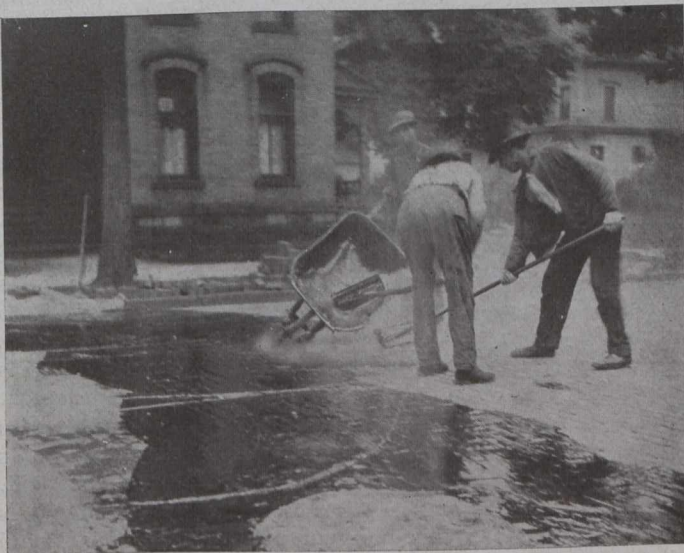
Fig. 1.—Finishing Mastic Filler on Brick Pavement.
