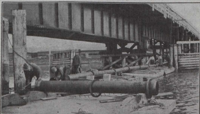
Fig. 14.—13-in. Flexible Pipes on Pontoons Before Lowering on River Bed.
