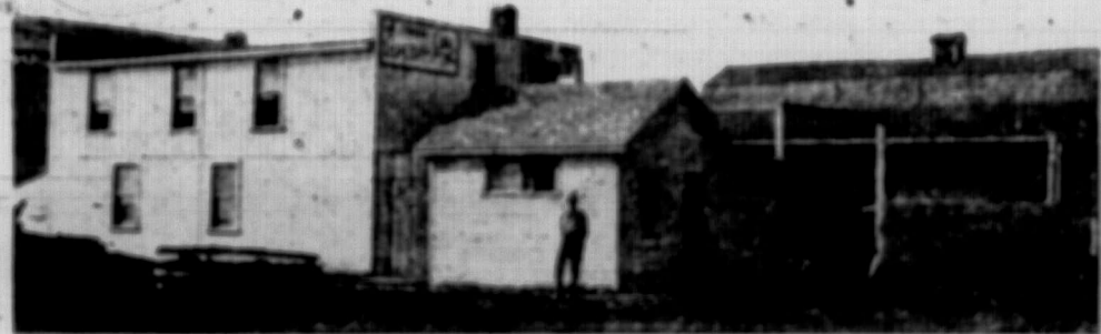
The Office and Yards of the Blackie Co-operative Association, Ltd., which does a Flourishing Lumber Trade
