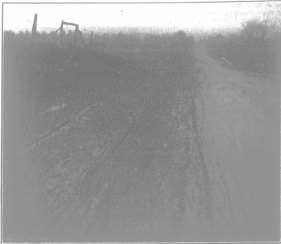
No Ditches on Either Side to Let Water Away.
