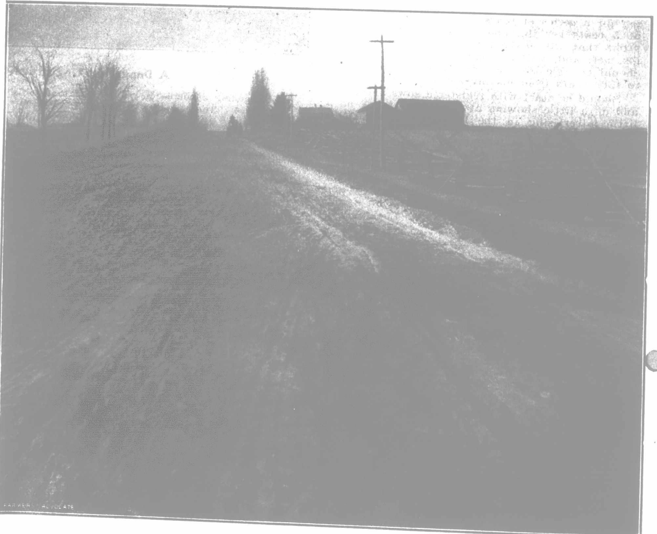
The King's Highway Drying Out.
