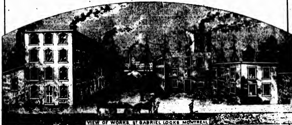
VIEW OF WORKS ST GABRIEL LOCKS MONTREAL
