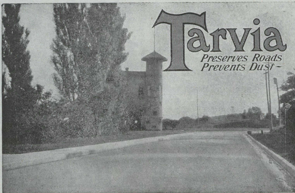
Westmount Boulevard, Westmount, P.Q. Constructed with "Tarvia-X" mixed method.
