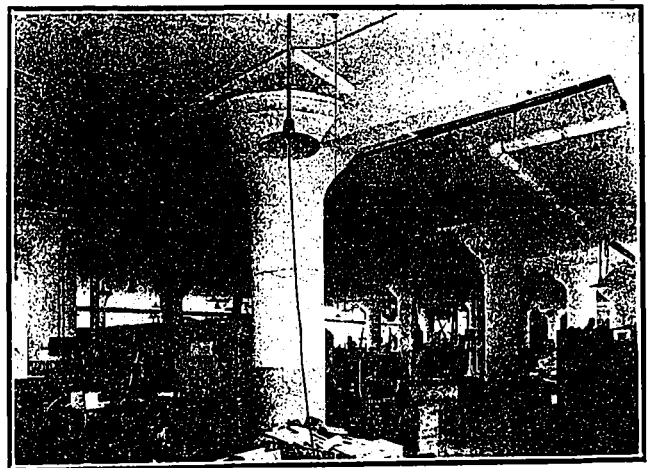
INTERIOR VIEW, SHOWING TYPE OF COLUMNS.
