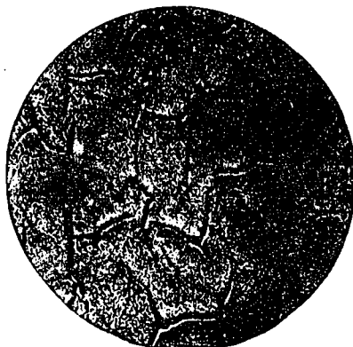
Figure 3.—Zinc oxide paint showing cracked condition.
