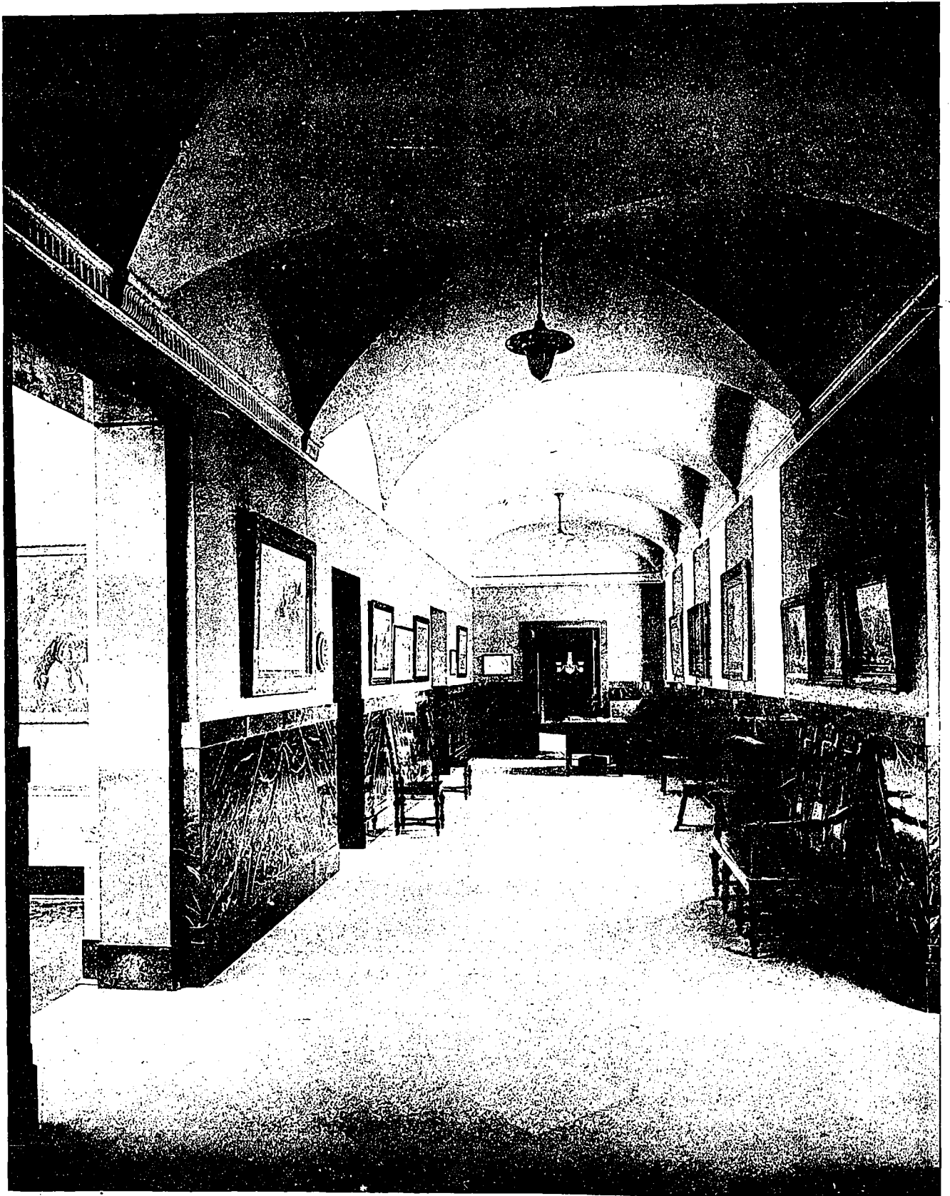
THE ART MUSEUM OF TORONTO. PRESENT ENTRANCE CORRIDOR LEADING FROM "THE GRANGE" TO COMPLETED PORTION OF GALLERY. DARLING & PEARSON, ARCHITECTS.
