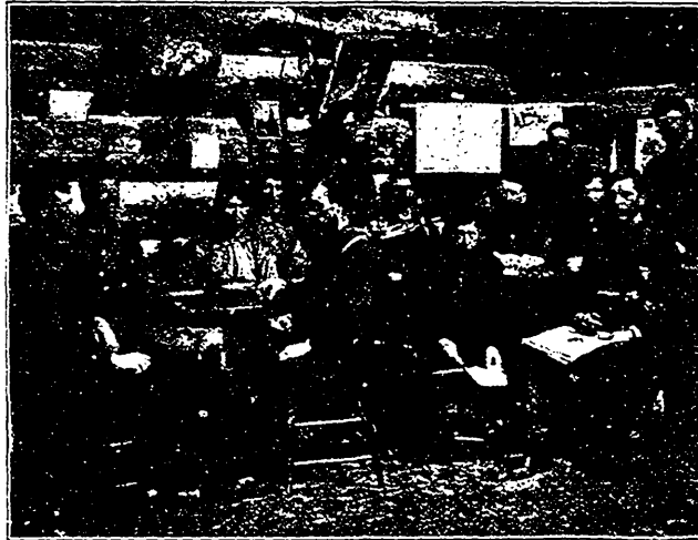
INTERIOR OF ONE OF PARRY SOUND CO.'S READING CAMPS.
