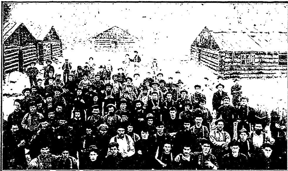
LOVELAND AND STONE'S CAMP NO. 1, READING ROOM IN BACKGROUND.
