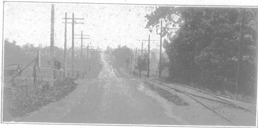
Kingston Road, Scarborough Township, Ontario. Treated with "Tarvia-B" in May, 1918. Toronto & York Roads Commission.
