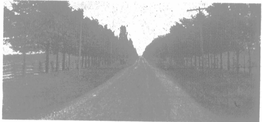
Kennedy Road, Scarborough Township, York County, Ontario. Tarvia filled macadam.
