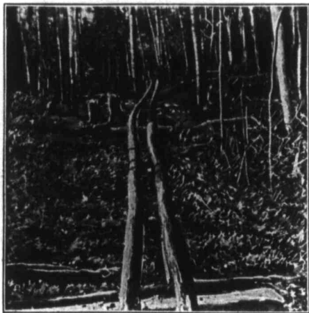
Tramway from No. 1 shaft to dock, length 340 feet.
