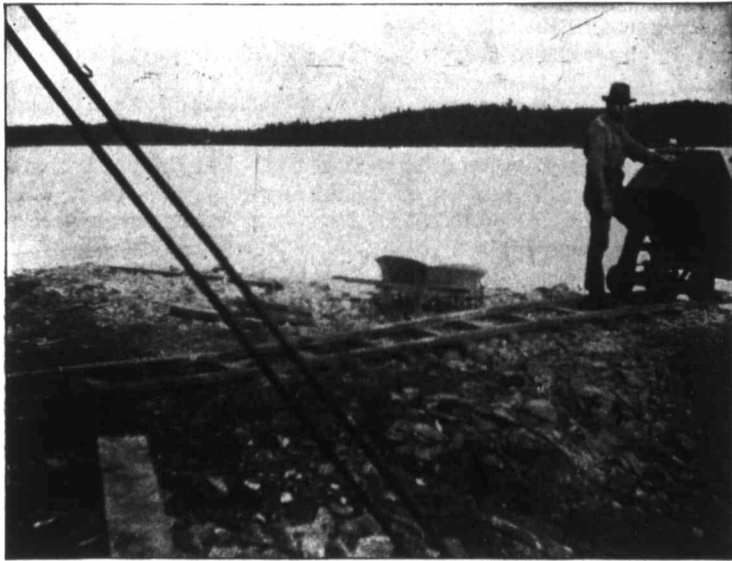
Miner dumping waste rock into Grace Bay from Tunnel.
