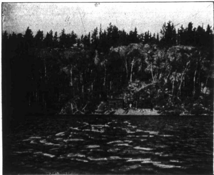
Tunnel Hill, showing Tunnel from a distance. One hundred and fifty-eight feet of work done in this Tunnel, March, 1903.
