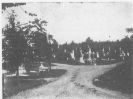
General View looking from Spruce Avenue.
