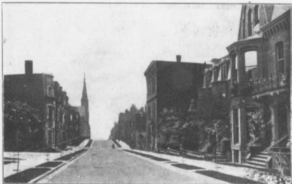
The Boulevard, Germain Street, looking South from Horsfield Street.
