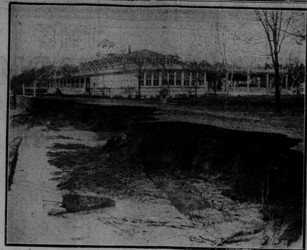
The high east winds of Saturday and Sunday last raised a storm on the lake that has done a good deal of damage along the shore. The beaches at the east end of the city have suffered considerably, and the island shore has been to some extent eaten into. The above photo shows the damaged promenade at Scarborough Beach Park. The concrete retaining wall has entirely disappeared, and serious inroads were made in the park property.
