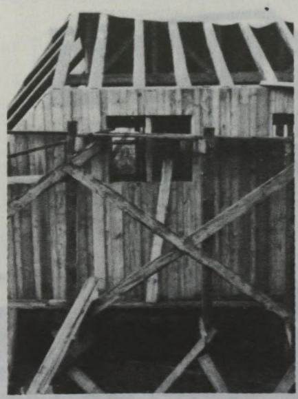
5 North wall bedroom window and roof framing, Waswanipi house.
