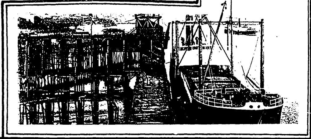
Loading coal from the huge Nanaimo bunkers
