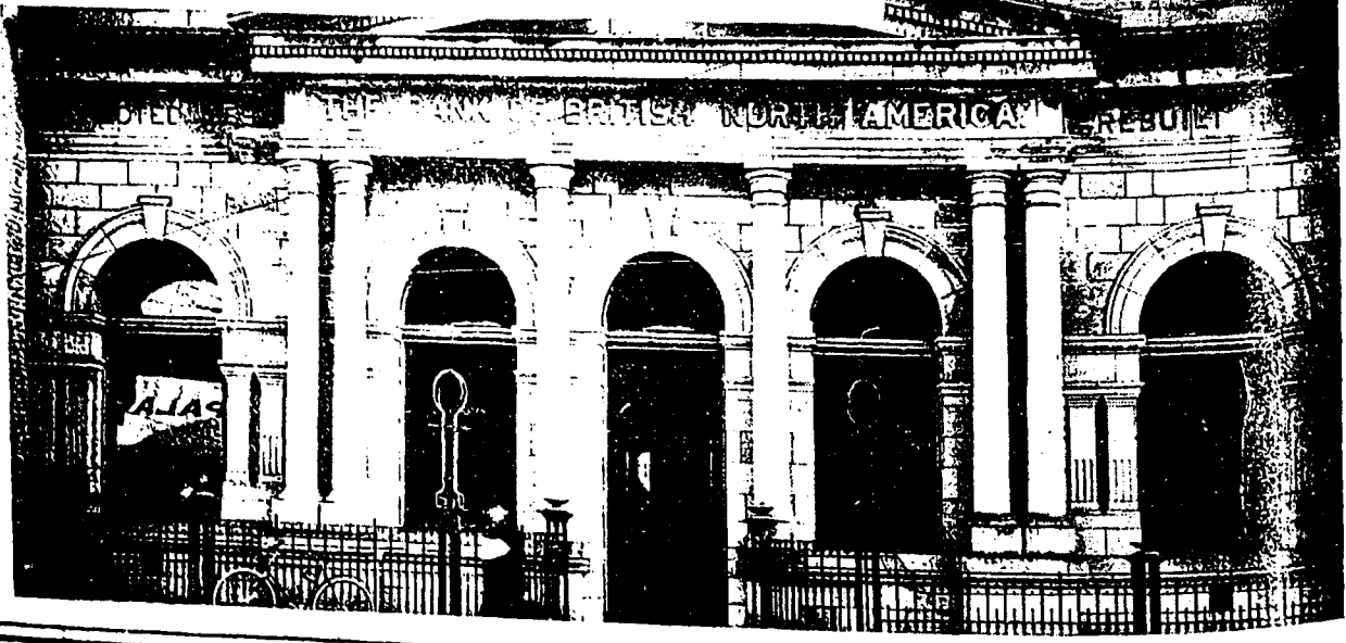
The building of the Bank of British North America, Victoria
