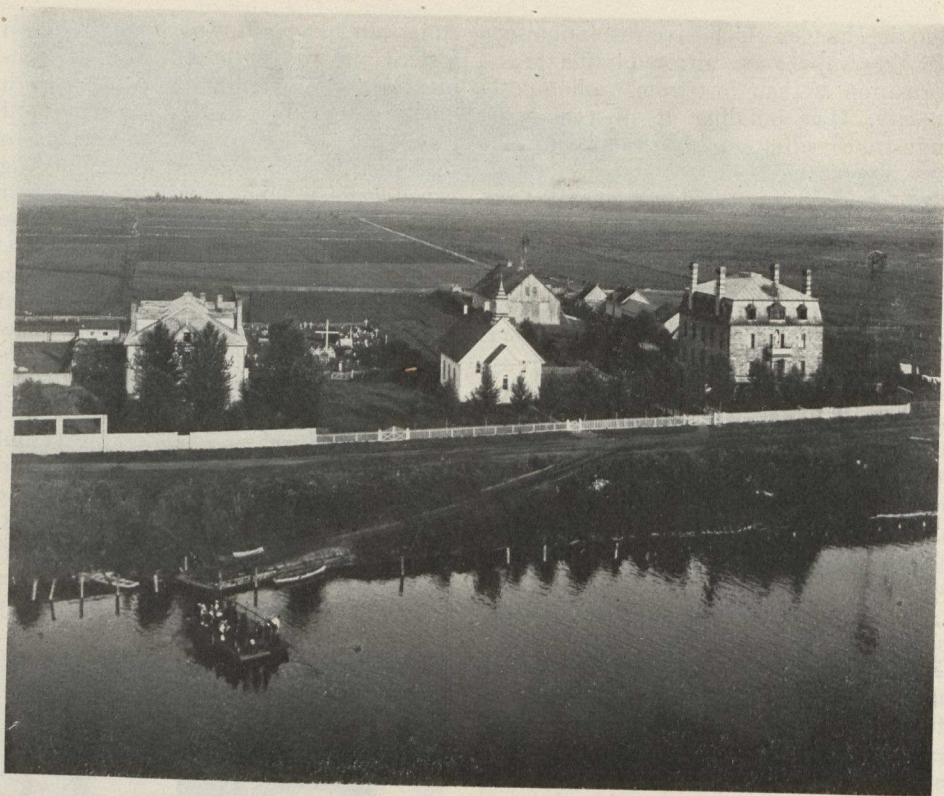
GENERAL VIEW OF R.C. MISSION
