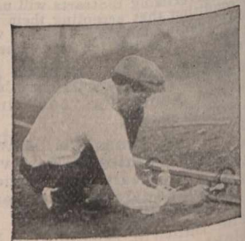
APPLYING THE SOLDER
