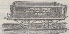
62—R. H.'s Patent Steel Goods Wagon, with Side Doors
