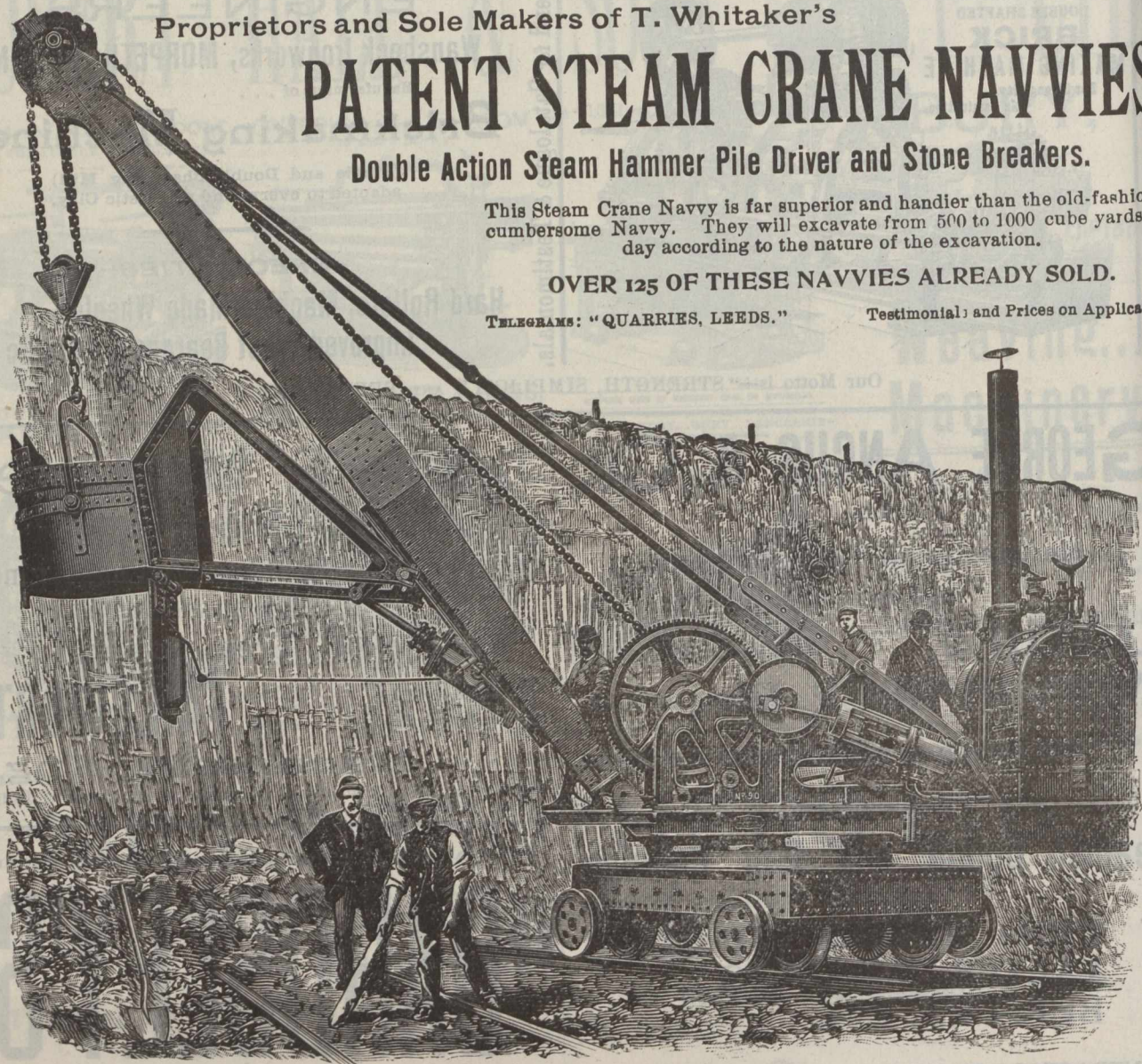
AS AT WORK ON THE MARSH LANE TUNNEL CONTRACT, LEEDS.
