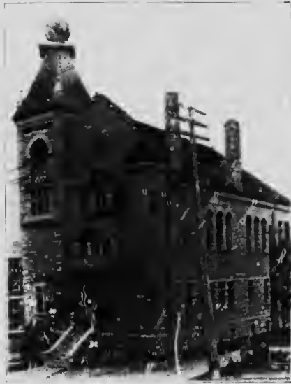
Onondaga Limestone. Municipal Buildings, St. Mary's, Ont.
