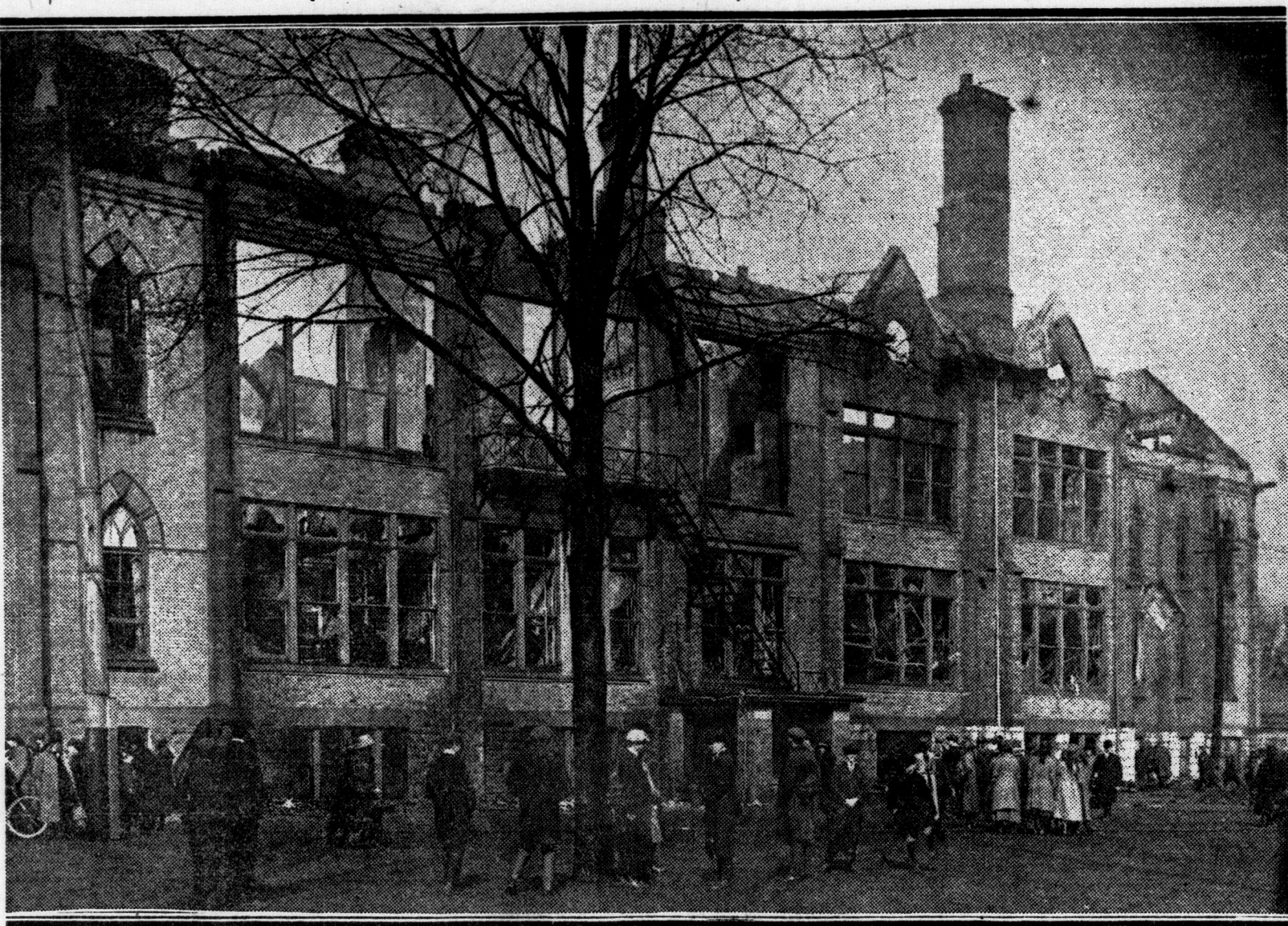
London Collegiate pupils viewing smoking debris this morning from east side of building, gutted by fire last night.
