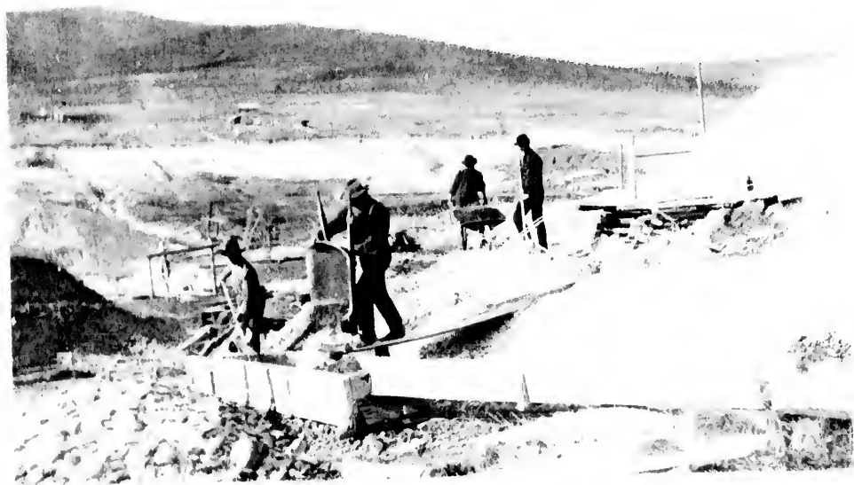
VIEW FROM DAM CONSTRUCTION
