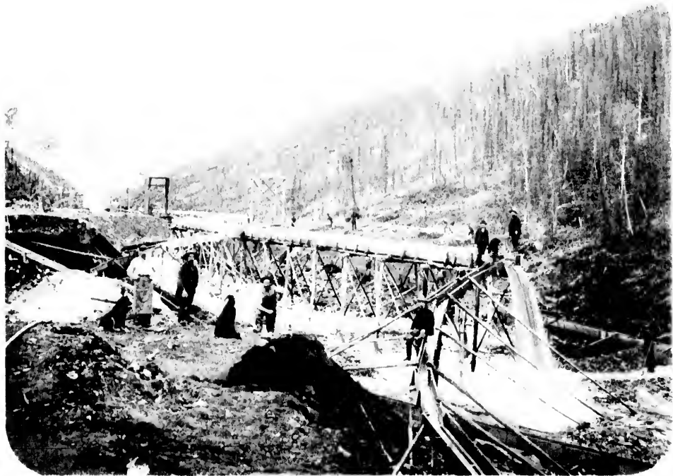
BRIDGE UNDER CONSTRUCTION
