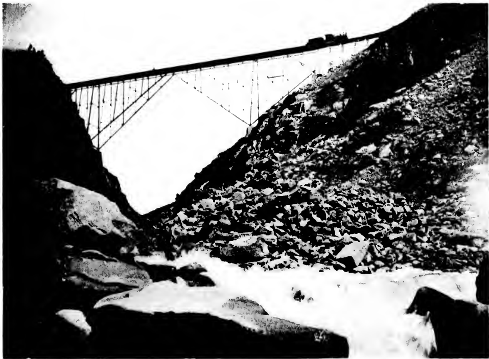
STEEL BRIDGE, SUMMIT OF WHITE PASS, ALASKA
