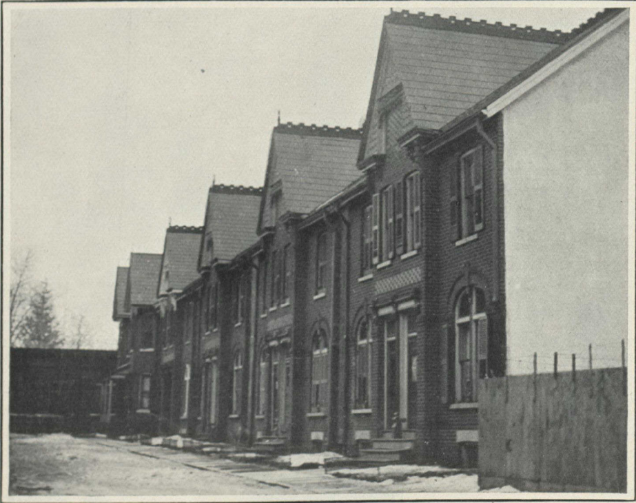
ROUGHCAST HOUSES, WITH BRICK FRONTS AND UNATTRACTIVE GABLES—A RESULT OF "BOOM" TIMES IN TORONTO
