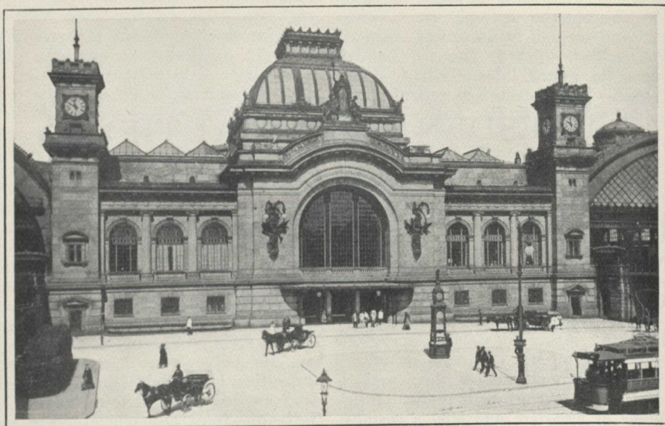
THE RAILWAY STATION, DRESDEN
