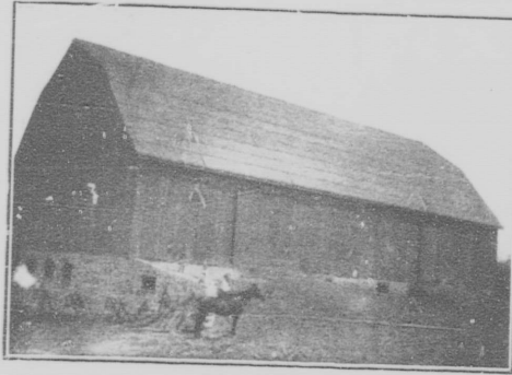
Reproduced Photograph of J. W. Young's Barn, Ryckman's Corners, Ont.
