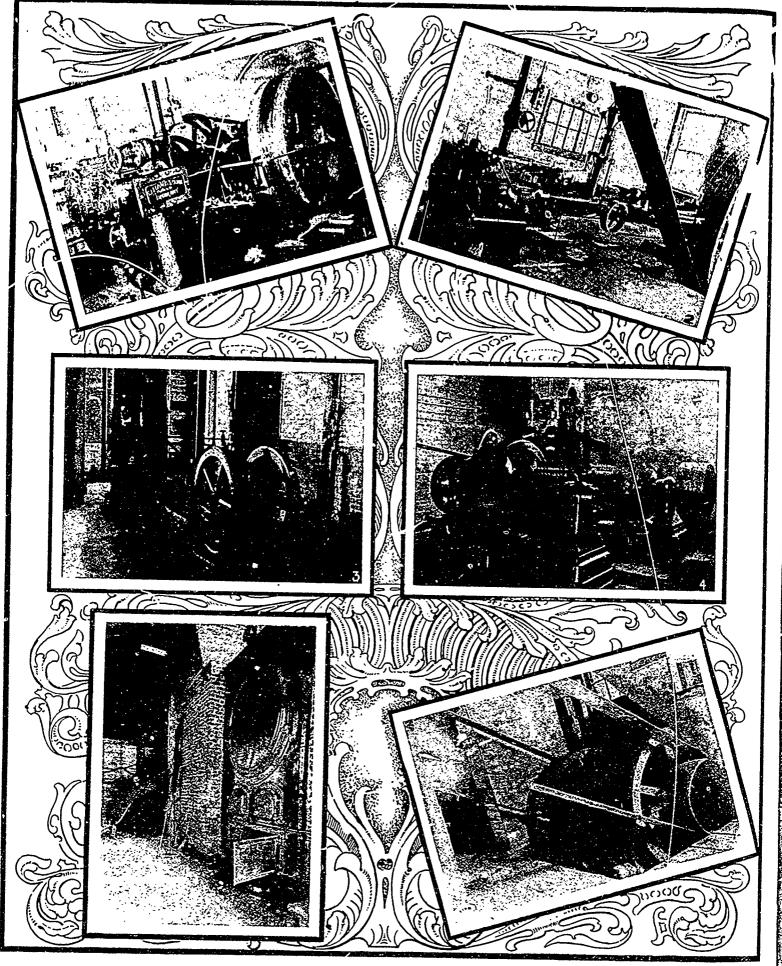
MINING AND MILLING PLANT OF THE INTERCOLONIAL COPPER CO. AT DORCHESTER, N.B. 1. Leonard Engine. 2. Laurie Engine. 3. Air Compressor at No. I Shaft. 4. Dynamo and Switchboard. 5. Boiler Room at Mill. 6. Ore Breaker and Rolls.
