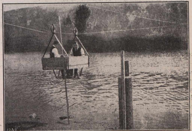
Fig. 8.—Cable Car and Gauge on Elbow River at Calgary.
