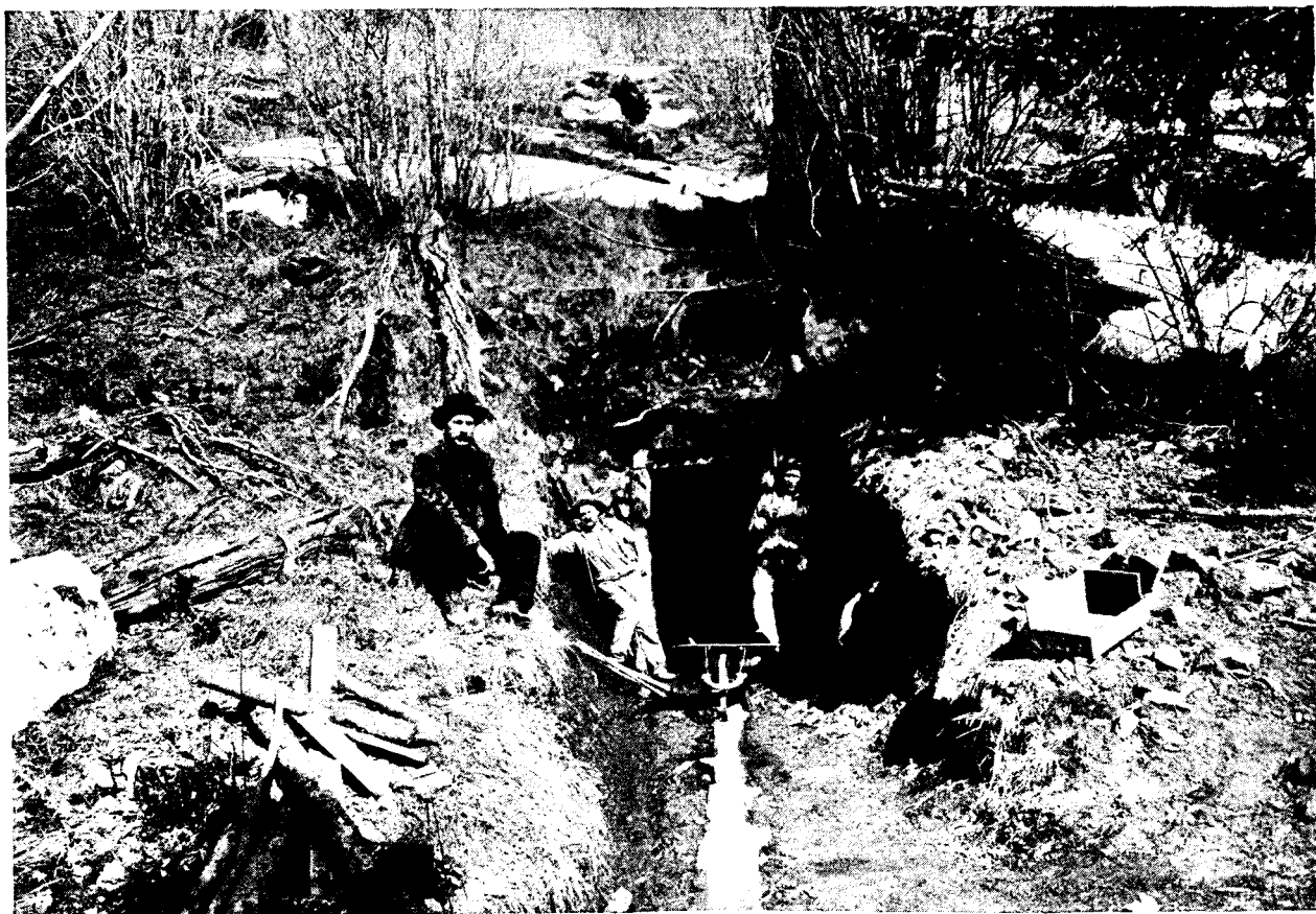
Entrance to Tunnel of Shannon and Dolphin Mine, Camp McKinney.
