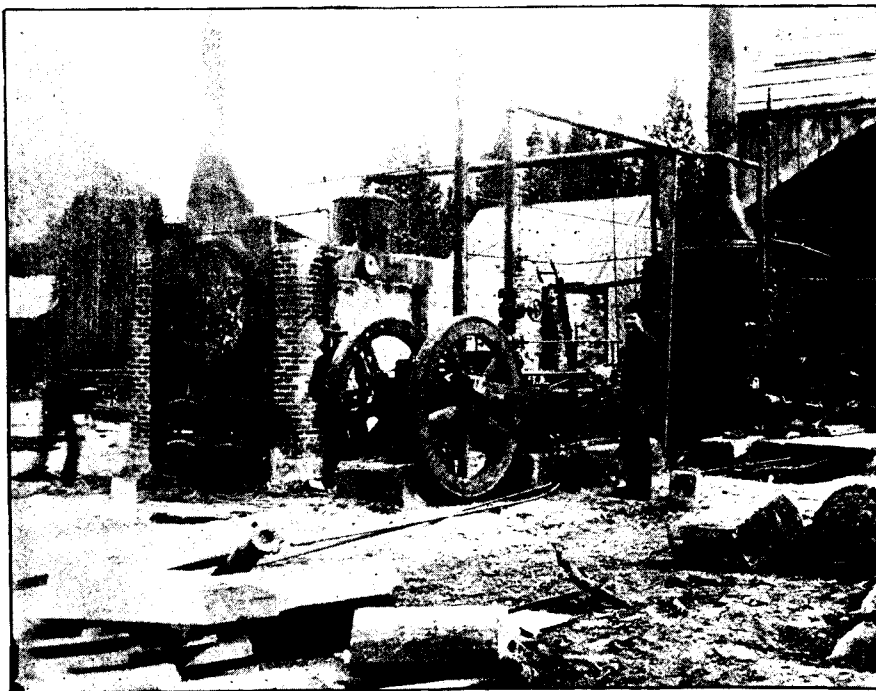
The Minnehaha Compressor.
