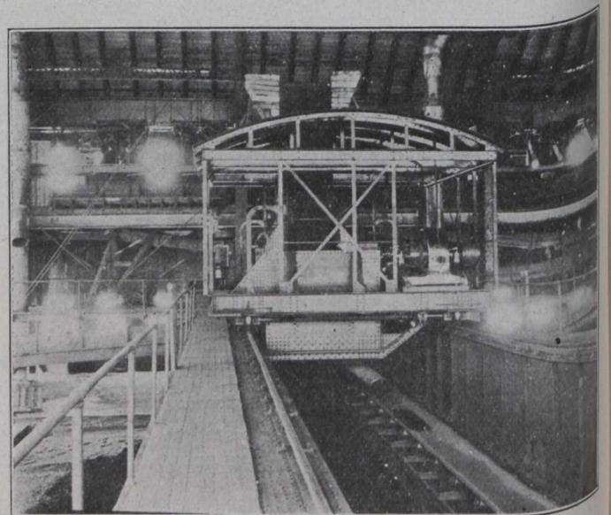
Washed Coal Elevator. The suspension rods and tables appear in the upper background. Dominion Iron and Steel Co., Limited, Sydney, N.S.
