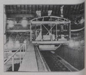
Washed Coal Elevator. The suspension rods an d trengle of tables appear in the upper background. Dominion Iron and Steel Co., Limited, Sydney, N.S.
