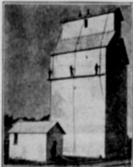
The Standard Elevator built by the Gillespie Elevator Construction Company.
