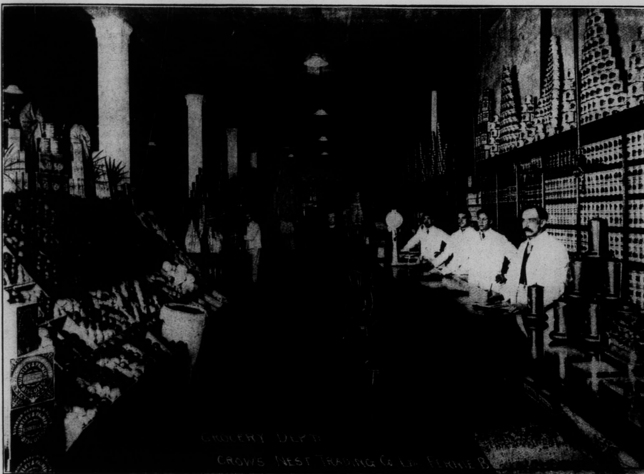
An Interior View of the Grocery Department of the Crow's Nest Trading Co., Fernie, B.C., With Some Good Ideas on Interior Arrangement.
