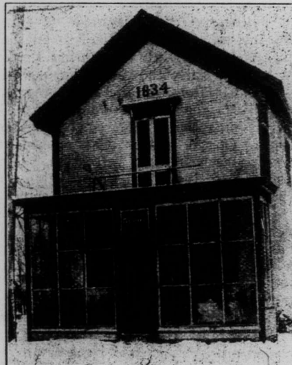
Store of Dyer & Son, Sutton, Que., Which Was Built 75 Years Ago.
