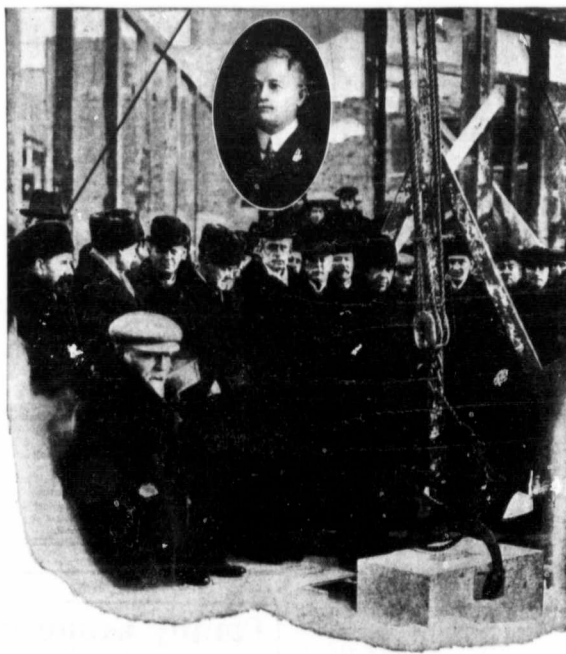
The laying of the Cornerstone of the Winnipeg Industrial Bureau's New Permanent Exposition Building, by His Honor, The Lieutenant Governor of Manitoba, on Dec. 30th, where the product of Winnipeg factories and labor will be exclusively shown. The insert is a photo of Lieutenant Governor D. C. Cameron, and in the front row facing reading from left to right are:—W. J. Bulman, Chairman of the Trade Expansion Committee of the Bureau; next the Governor; Major R. D. Waugh; F. W. Heubach, President of the Bureau; Ex-Mayor W. Sanford Evans; James Scott; and C. N. Bell, of the Winnipeg Board of Trade, in foreground.
