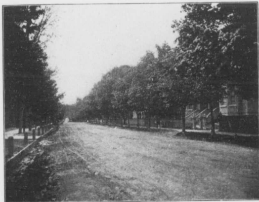
FROST STREET—LOOKING WEST
