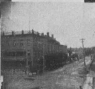
UNION ST. LOOKING EAST.
