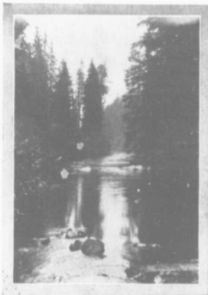
PROPOSED NEW SEYMOUR INTAKE AND DAM FOR STORAGE RESERVOIR. VIEW IS TAKEN AT TOP OF FALLS
