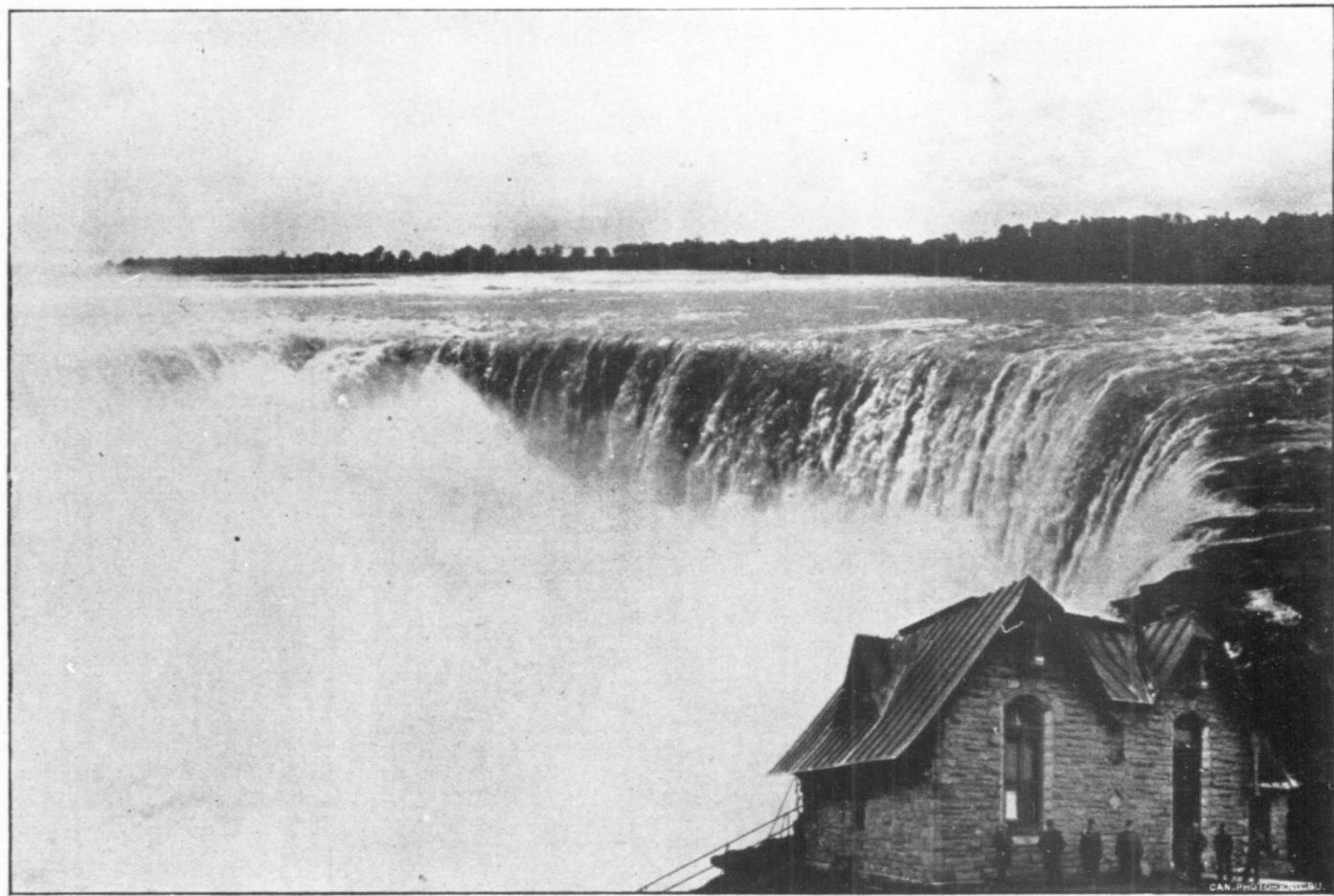
WATER WORKS PUMP HOUSE AND HORSESHOE FALL.
