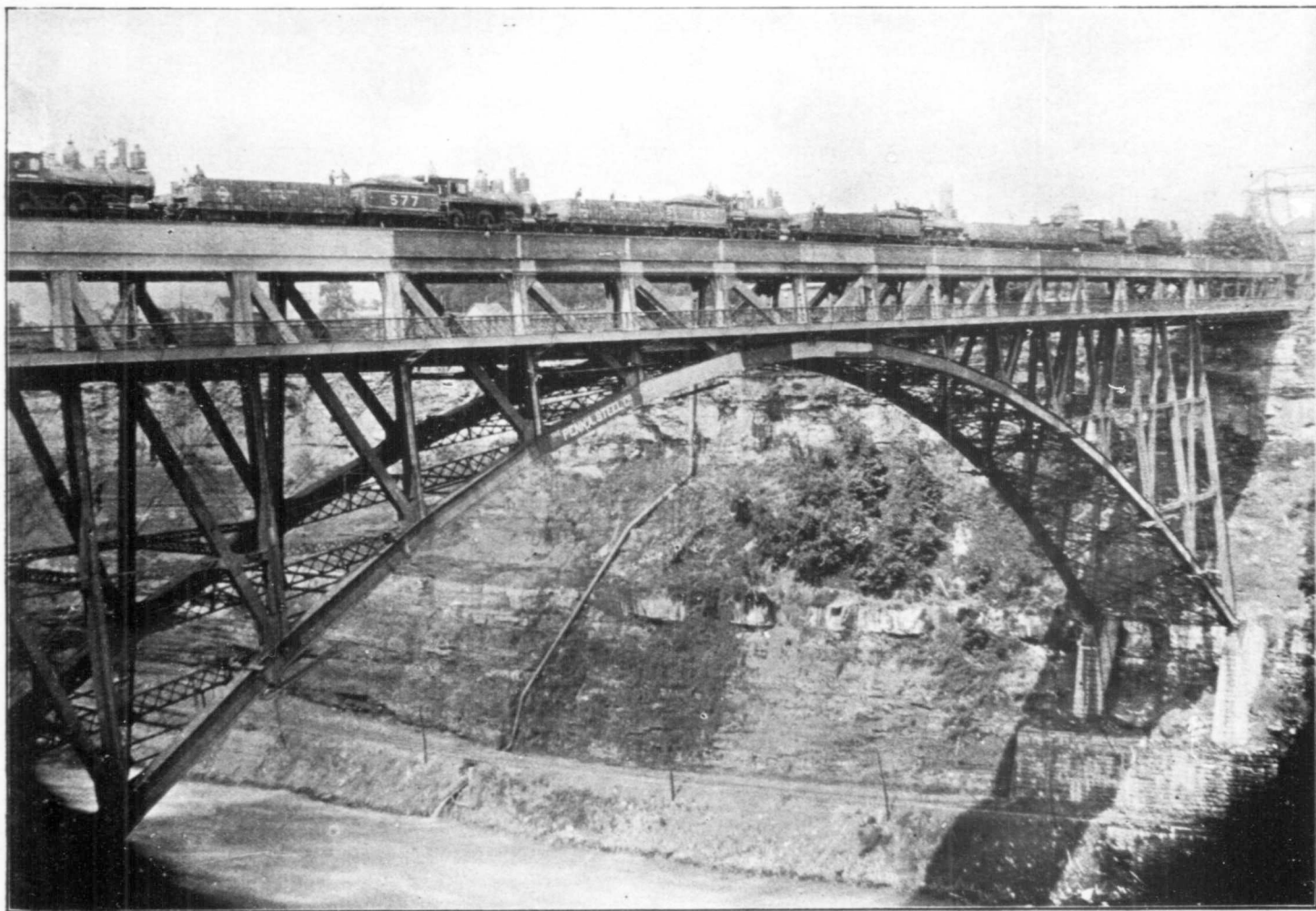
NEW STEEL ARCH BRIDGE.
