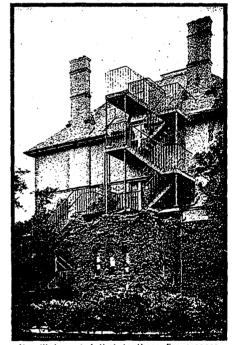
t will be noted that in these fire escapes erected in England, that they are really external iron staircases, having iron guardrails; gangways to roof; balconies and foot bridges. The above is a fire escape on a private residence.
