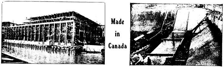
Bostwick-Brown Hardware Co. Building, Toledo, Ohio. Walls and floor are 20 ft. below water level. "Medusa" Waterproofing used in basements.
