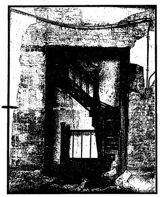
View showing interior stairway, New York catastrophe, where the charred wooden handrais and steps give evidence of how the flames leaped through the doorway and up the stairway, thus cutting off this means of egress from the building.
