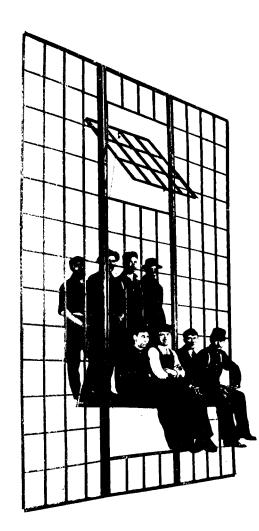
The muntins are deep and narrow, offering a minimum obstruction to the light. The joints are not weakened in any way by cutting or punching.
