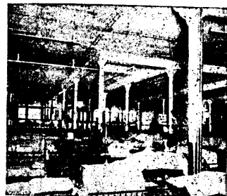
After Luxfer Prisms Installed.
