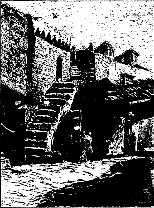
OUTSIDE STAIRS TO FLAT ROOF.
