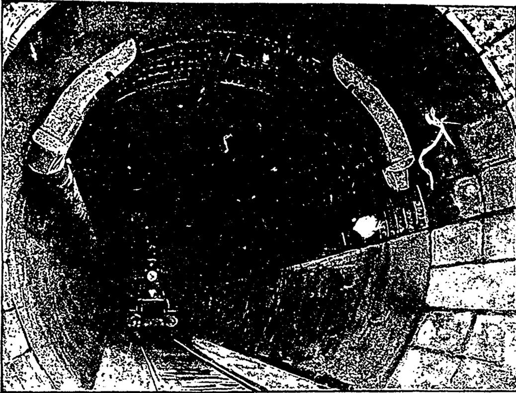
the tunnel proper is 6,025 feet, and of the portals that form the approaches 5,605 feet in addition, or more than two miles in all, being the longest submarine tunnel in the world. It is a continuous iron tube 19 feet 10 inches in diameter, put together in sections as the work of boring proceeded, and firmly bolted together, the total weight of iron aggregating 56,000 pounds. The tunnel commenced in September, 1888, was opened for freight traffic in October, 1891, and passenger trains
