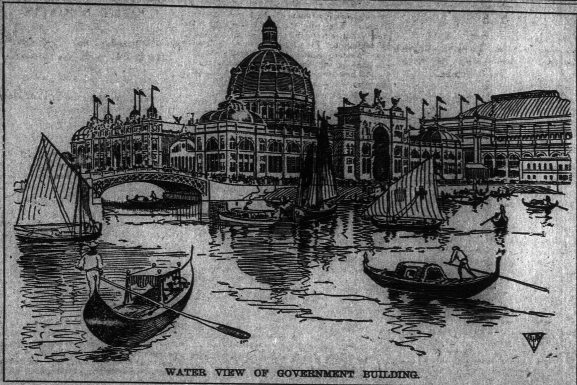
WATER VIEW OF GOVERNMENT BUILDING.
