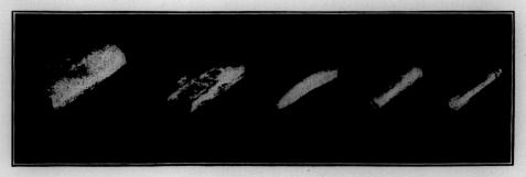
Five phases in the manufacture of an amber mouthpiece. On the left is the rough hewn lump, fresh from the mines in the Baltic. Number two, the same piece cut in two. Then a well-chiselled lump. Next we see the mouthpiece taking tangible shape, and finally ready and waiting to be screwed into the meerschaum pipe.
