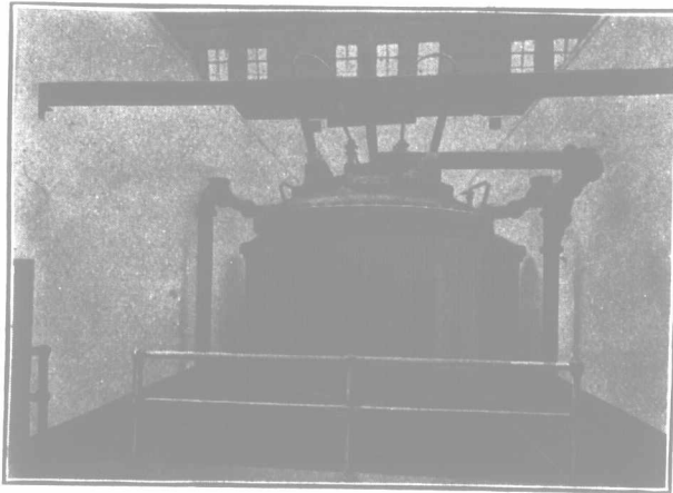
Transformer Unit, Ontario Power Co.
