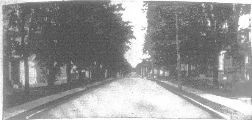
Wellington Street, Stratford, Ontario, "Tarvia-X" pavement constructed in 1913. Surface treated with "Tarvia-B" 1917.
