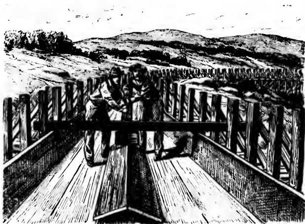
FLUME BUILDING. SPRINGING IN THE BOTTOM PLANK.
