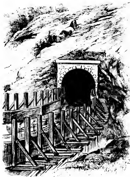
TUNNEL PORTAL, SAN DIEGO FLUME.
