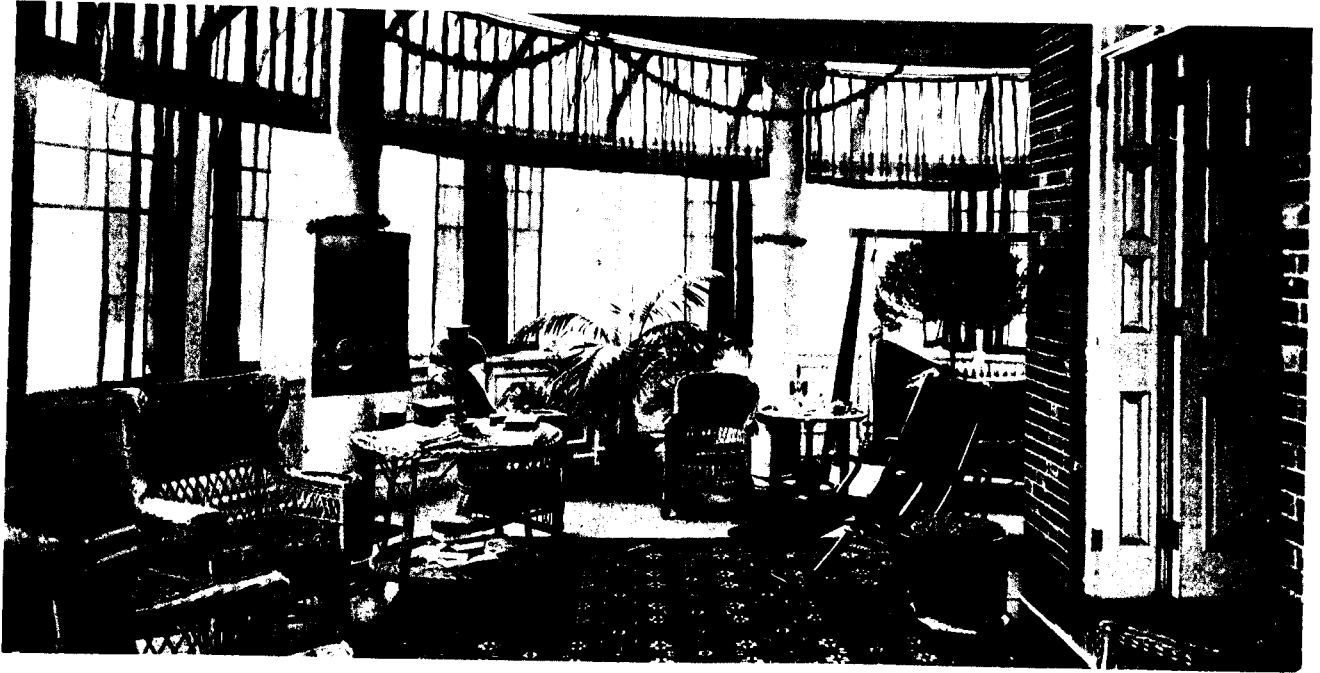
Interior of an Enclosed Porch at Wilmington, Del.
