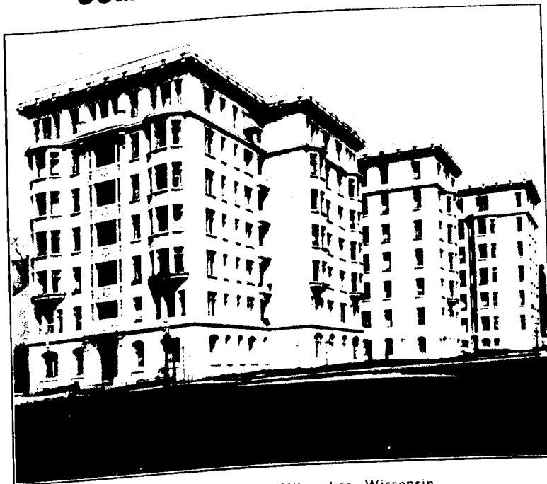
Cudahy Apartments. Milwaukee, Wisconsin.
