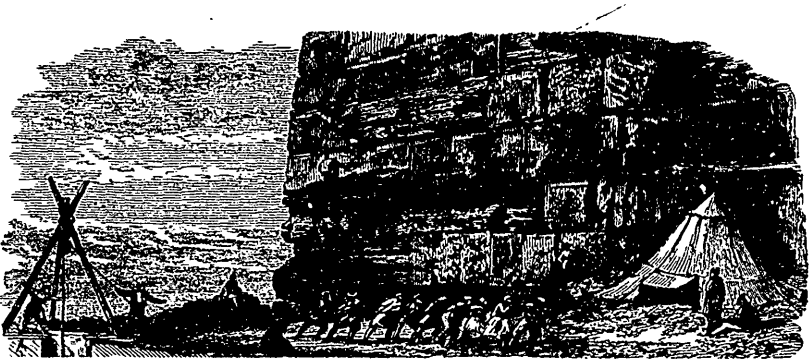
EXPLORATION BENEATH THE WALLS OF JERUSALEM.
