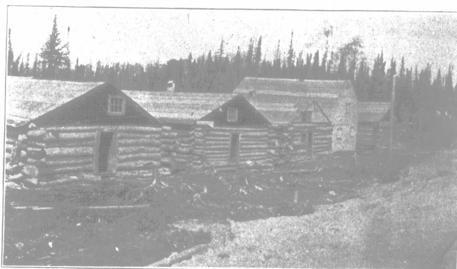
Familiar Architecture in the North. Construction camp on the road to Porcupine.
