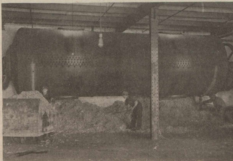
The cooked rags are removed from the boiler and carted to the washing engines. The man at the right is seen adjusting the waste liquor pipe.
